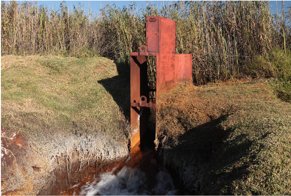
Fig. 5 Abandoned flow gaging station at the end of the natural wetland area of the Tweelopiespruit. Corrosion from the initial acid mine drainage and gypsum precipitates from the treated mine water can be seen at the flow gages' outflow. Photograph: Christian Wolkersdorfer.
