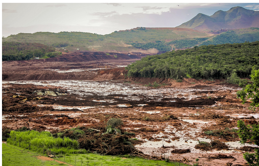
Fig. 8 Mudflow from the collapse of the B1 Dam at Córrego do Feijão Mine, Brumadinho City region, Minas Gerais State, a tailings dam failure that caused severe social and environmental impacts. Photograph: Isis Medeiros.
